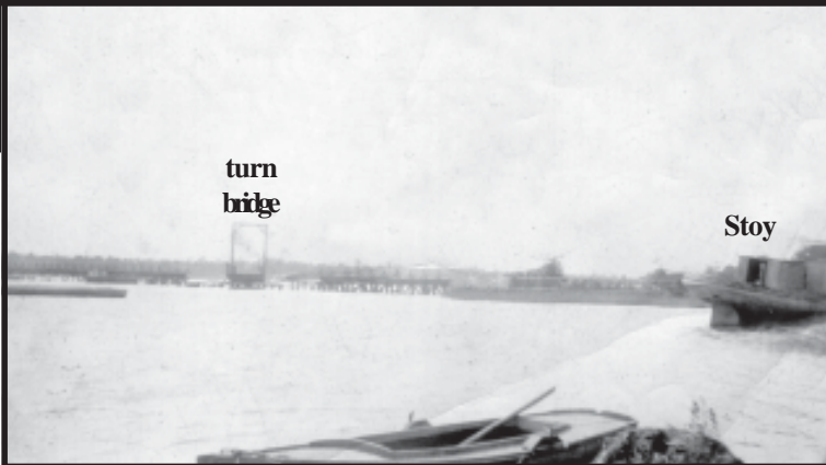
The first Wading River bridge was a turn bridge that rotated to open. The Stoy can be seen beached to the right of the bridge. (Photo courtesy of Steve Eichinger.)
