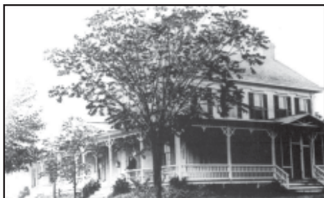
The French house on Main Street in Port Republic. (Photo courtesy of Port Republic 2000 Booklet)
